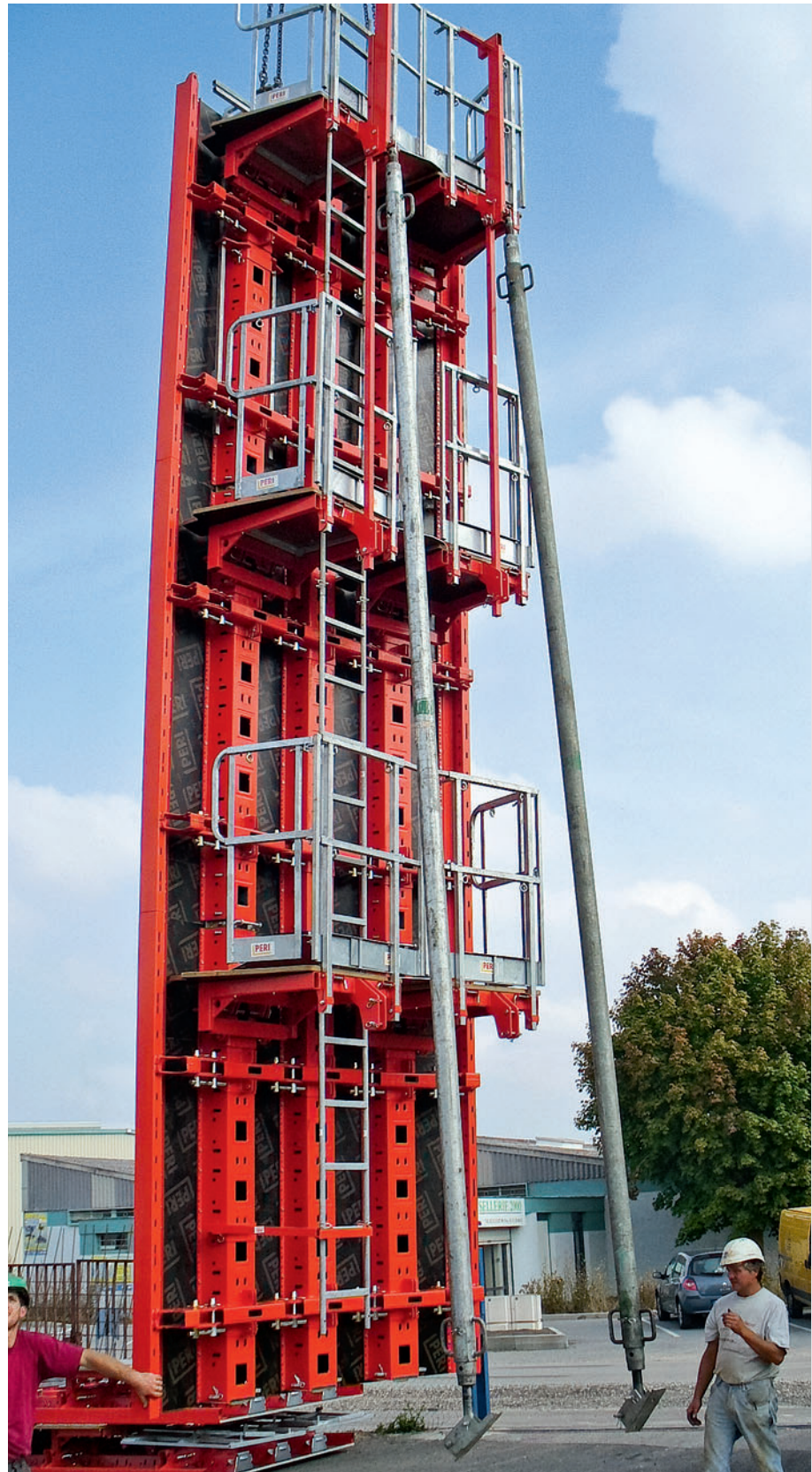
Complete element with platforms, access ladder and push-pull-props being moved to its place of use.
