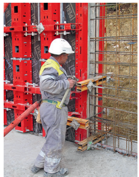
Conventional stopend formwork is mounted with walers and stopend ties.
