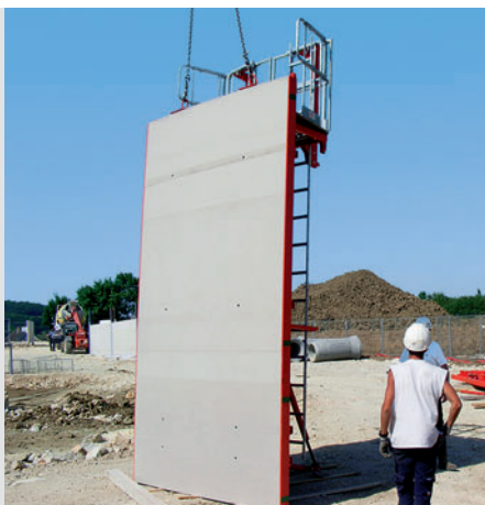
Using the RUNDFLEX Plus-2 results in high-quality concrete surfaces and a uniform curvature.
