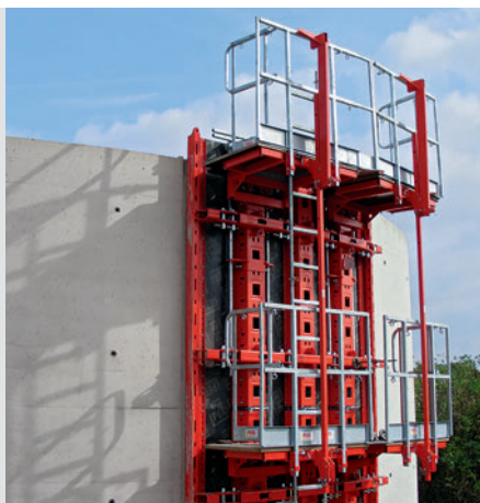
Formlining screwed on at the rear leaves no impressions on the concrete surface.
