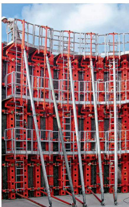
Formlining screwed on at the rear leaves no impressions on the concrete surface.
