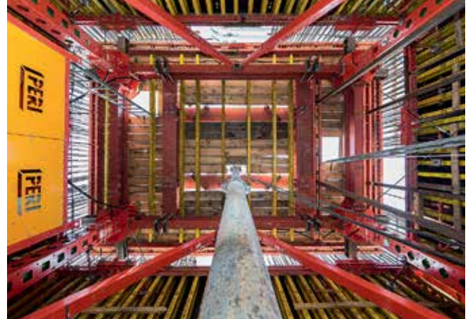
The ACS Core 400 ensured that the construction team was able to meet the extremely tight schedule.
