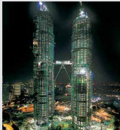
1994 Petronas Towers, Kuala Lumpur, Malaysia (ACS, VARIO GT 24)
