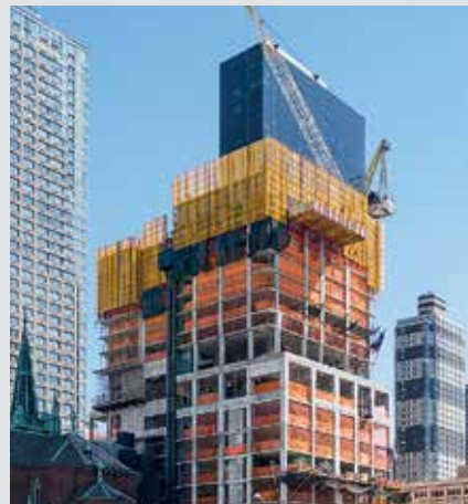
2015 555 Tenth Avenue Residential and Office Complex, New York, United States (LPS)
