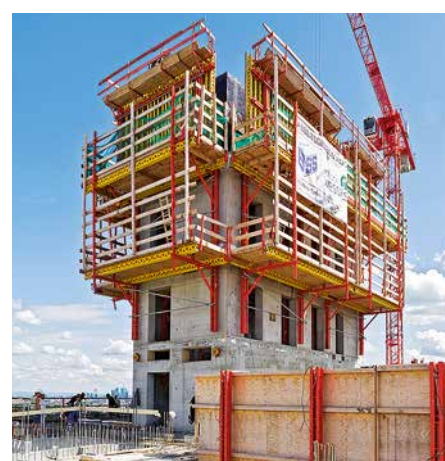
The RCS Rail Climbing System used as formwork scaffold for the building core and as a climbing protection panel on the facade.
