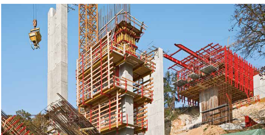
Another typical area of application for the RCS Rail Climbing System is bridge piers.
