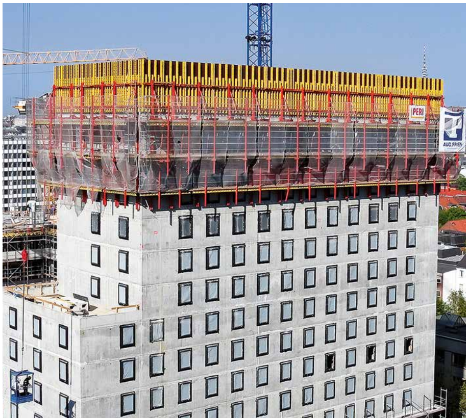
The RCS Climbing Formwork with continuous high side protection provides safe working areas at great heights.
