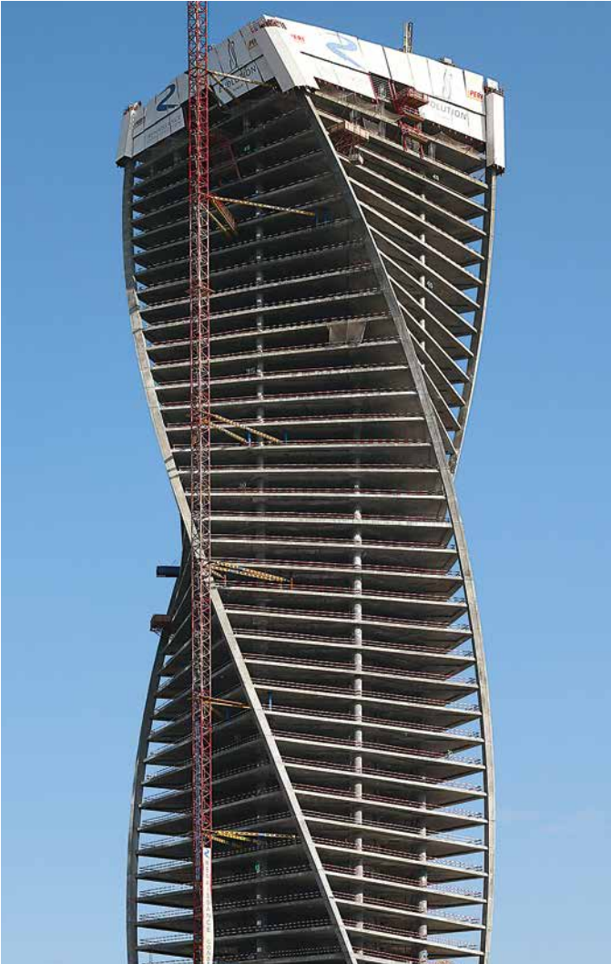
With a 150° rotation, the Evolution Tower twists its way upwards into the Moscow sky reaching a height of almost 250 m. Inclined and crane-independent climbing RCS Protection Panel Units provide a very high level of safety.
