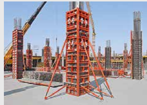
Column Formwork
