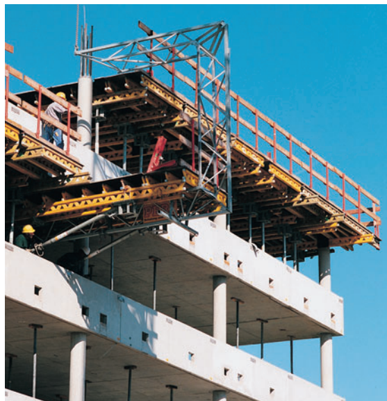
Vertical moving of PERI slab tables.
