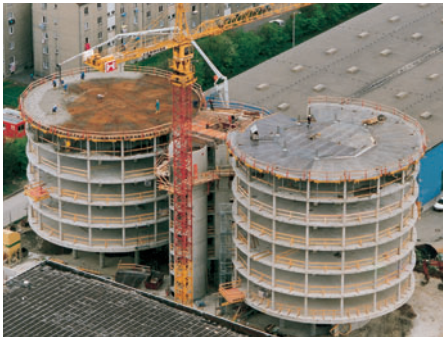
Trapezoidal-shaped UNIportal slab tables for a circular office building.
