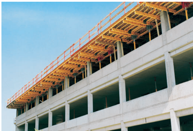
Cantilevered PERI UNIportal edge tables with guardrails.
