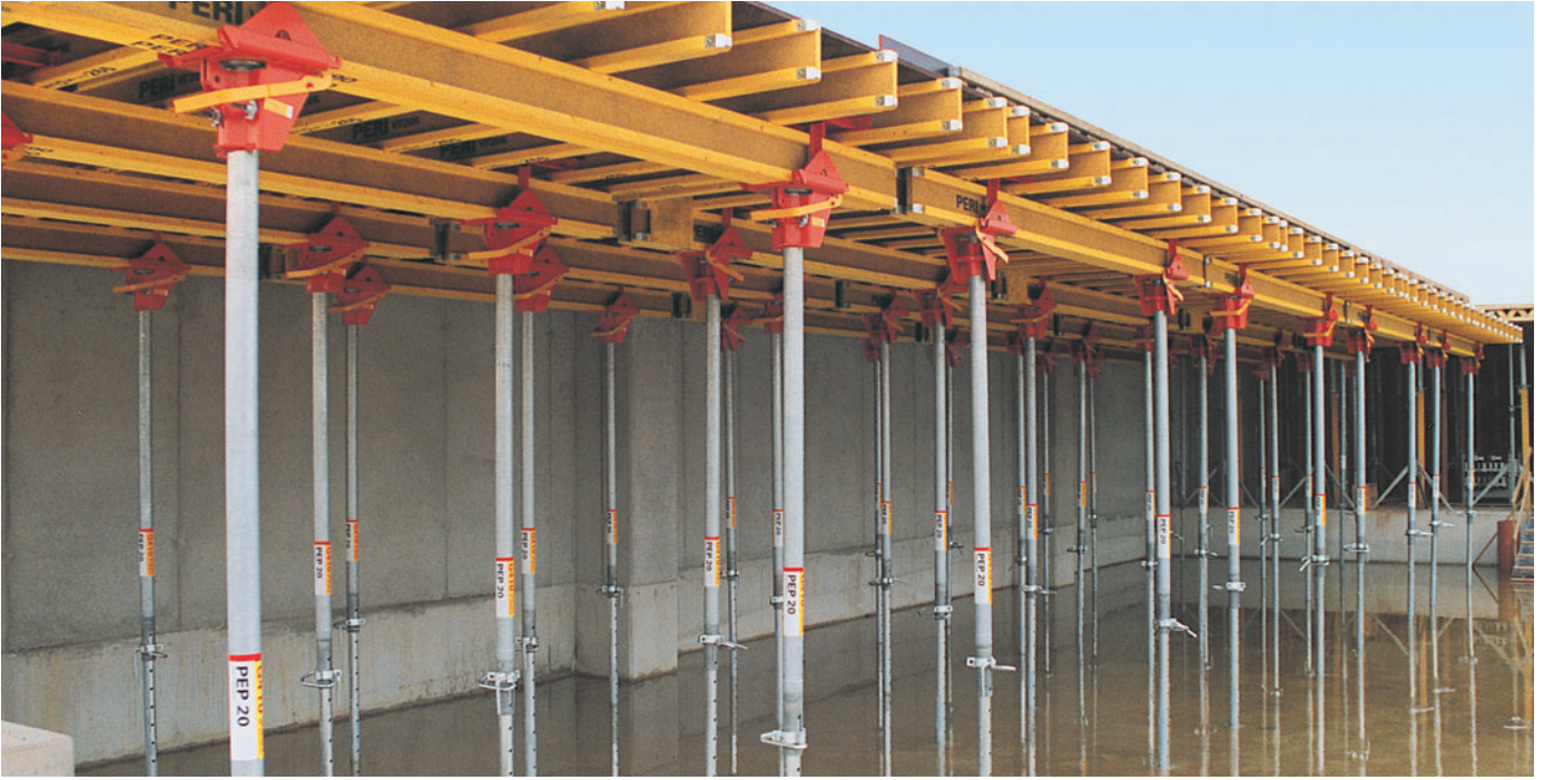
PERI Table Modules VT 250 / 265 x 400 used with PEP 20 props for industrial building.
