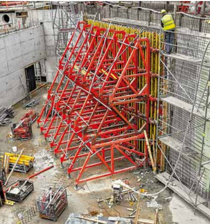
Force is safely and reliably transferred at all connection points of the SB-A0, A, B and C.
