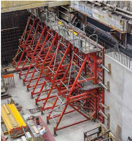
The required working platforms are correspondingly attached to the respective formwork system.
