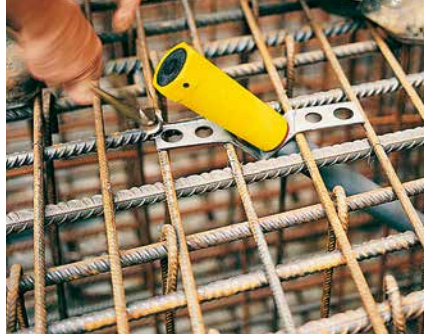
With the V-Tie Holder, as a lost part, an exact alignment of the Tension Anchor to 45 ° is possible.
