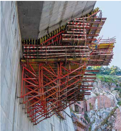
Brace Frames and system components taken from the VARIOKIT Engineering Construction Kit form large-sized platforms up to 8.75 m wide.
