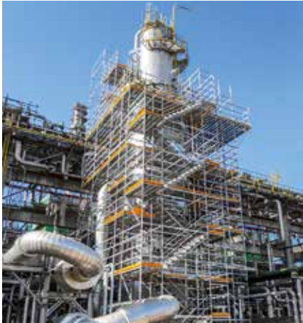
PERI UP Flex Stairs with closed decking areas can be flexibly integrated into the scaffolding solution to ensure safe access.
