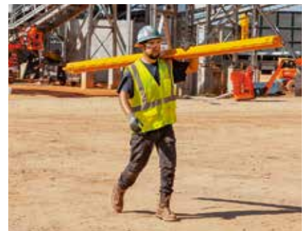
Due to the low weight and special design, the toeboard can be conveniently stacked and transported by hand.
